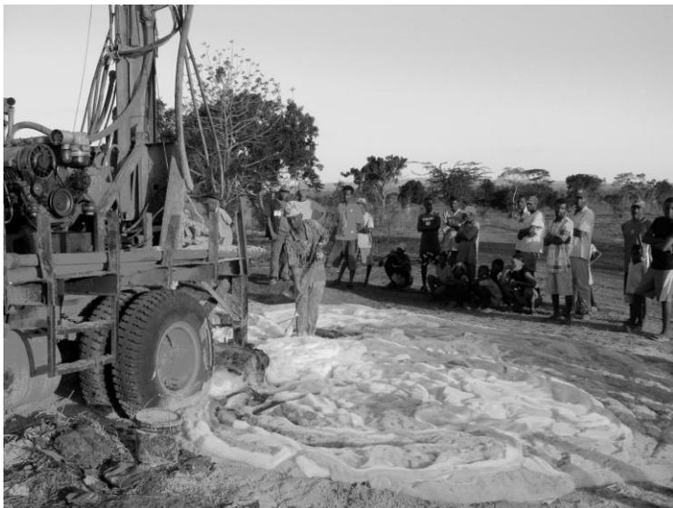
The community of Deux Baleins Nord watches as a well is drilled using foam with the converted rotary air hammer rig.
