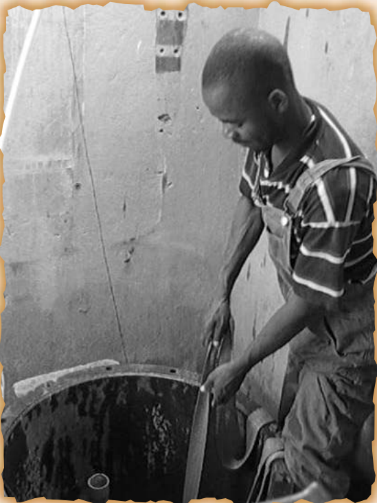
HAITI OUTREACH EMPLOYEE ADERBAL NORVIL WORKING TO CLEAN OUT AN IRRIGATION WELL ORIGINALLY DRILLED IN THE 1960'S
