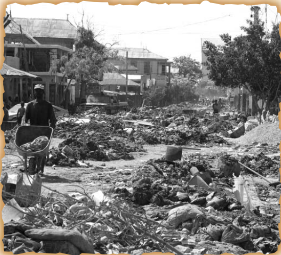
MUD AND DEBRIS PILED HIGH, BLOCKING THIS STREET IN GONAIVES SHORTLY AFTER THE CATASTROPHIC FLOODS BROUGHT ON BY HURRICANE JEANNE IN 2004.
