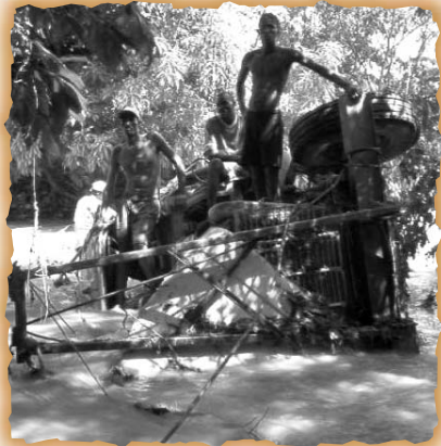
HAITI OUTREACH EMPLOYEES TRYING TO SALVAGE WHATEVER PARTS THEY CAN FROM THE TOPPLED WELL DRILLING RIG AFTER IT WAS TURNED OVER AND WASHED DOWN THE RIVER IN A FLASH FLOOD IN APRIL.
